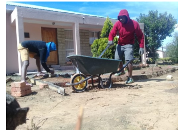
On site staff repairing the centre
